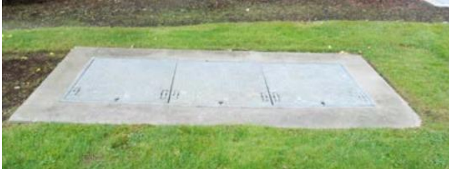
Typical Underground Distribution Feeder Cable Pull Vault
